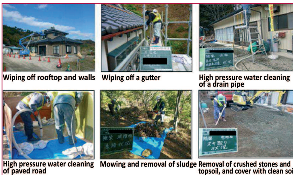
Fig. 9 - Demonstration of some decontamination methods utilized in the remediation works
